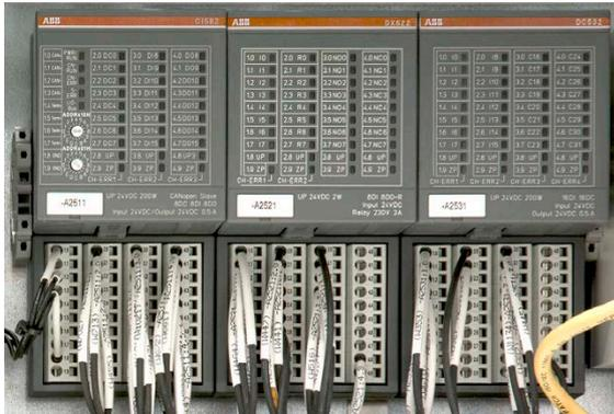
Figure 9-4 S500 I/O modules in a COU
