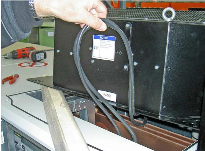
5. Put two pieces of square timber on the adjacent heat exchanger and place the removed heat exchanger on the timber.
