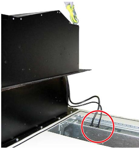
7. While lowering the heat exchanger onto the roof, pull the cables through the openings.
