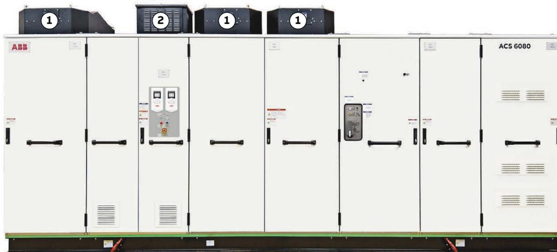
Figure 3-23 ACS6080 example drive with air-to-air heat exchanger
