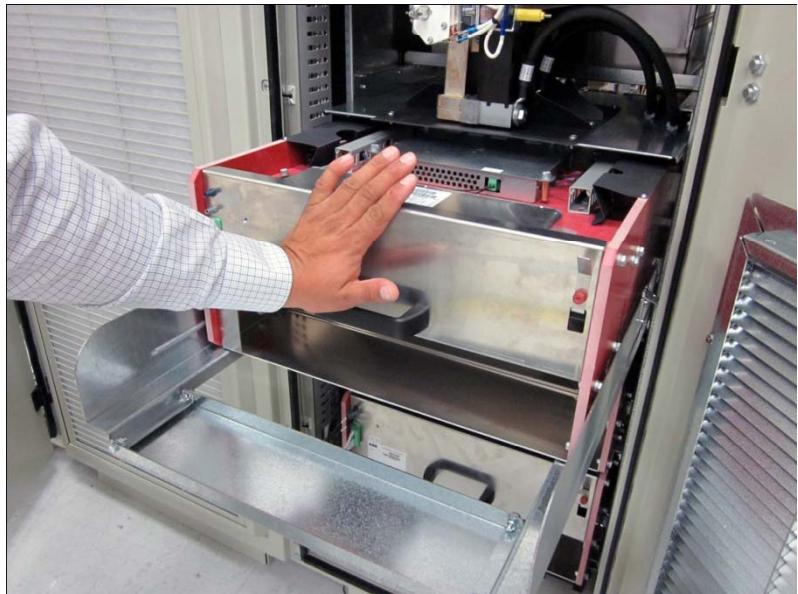
**NOTE:** Once in place, remove the phase capacitor shorting strip. Install strip on phase module that was removed.
