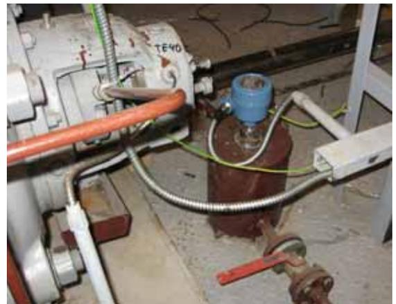
Figure 1: Rosemount 2120 Level Switch
